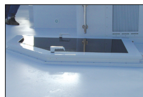
Ladderwell hatch, Proud coaming, Side view
