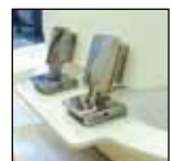
Flush surface hinge, Raised for teak overlay
